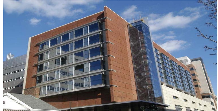
UMMS Hospital, Baltimore
