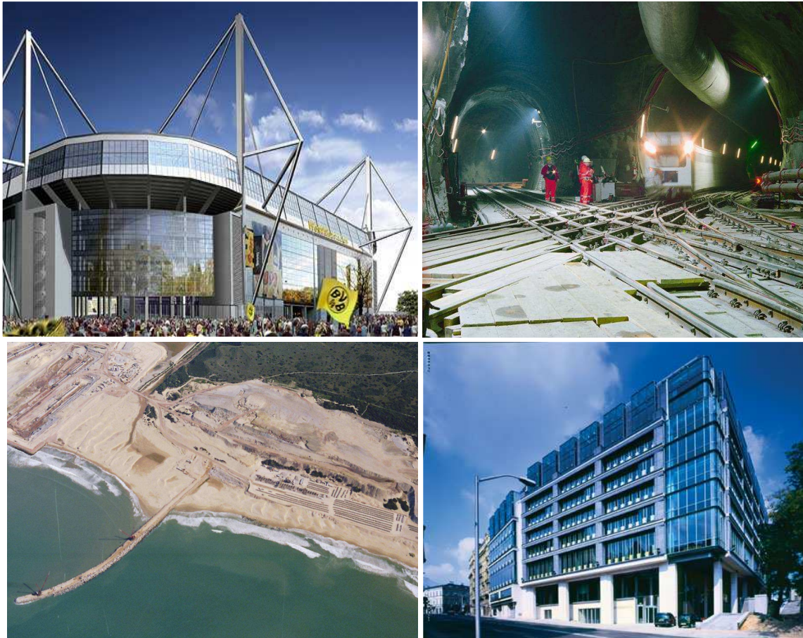
Top left: Westfalenstadion, Dortmund; Top right: St. Gotthard Tunnel, Switzerland; Bottom left: Port constructions Ngqura, South Africa; Bottom right: Stock Exchange Center, Warsaw
