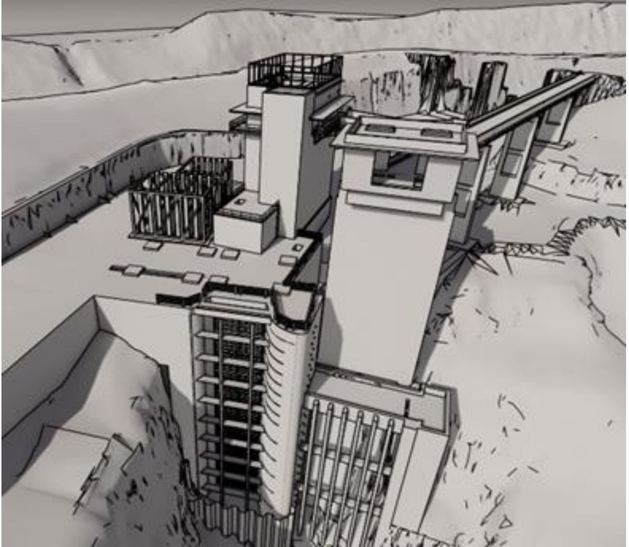
Graphic illustration of the additional water storage project at Howard A. Hanson Dam, showing the new fish passage facility intake and tower to the left of the existing regulating tower (right). Courtesy USACE
