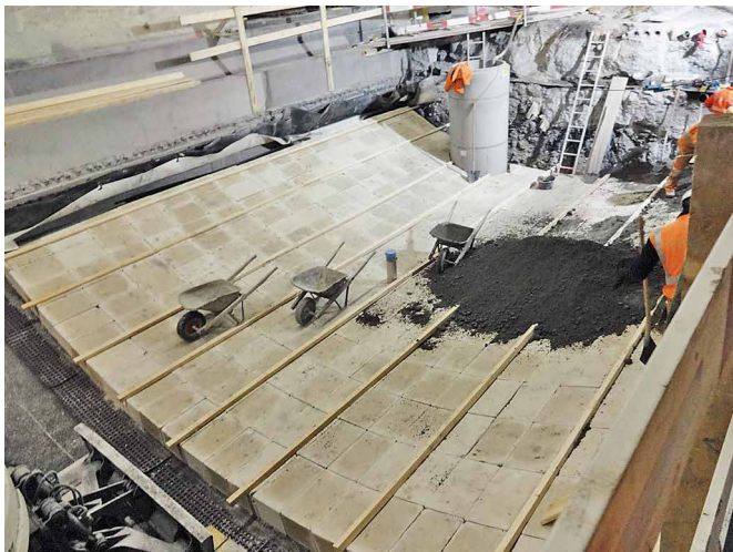
Fig. 3 Invert with yielding elements laid in position (photo from 9 May 2019)
