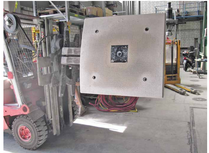
Fig. 8 Preliminary trials to test handling of Compex segments on the construction site
